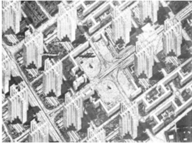
The Image shows an aerial view of the centre of the city and the cruciform skyscrapers. (4)
