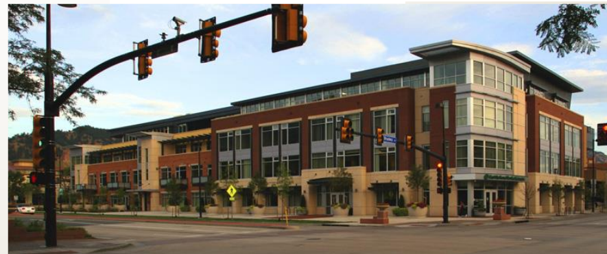
Mixed Use building designed OZ Architecture in Boulder, Colorado
